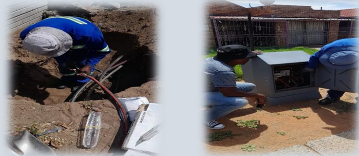
Photo2: Municipal staff repairing vandalised streetlights and kiosk in Retswelele & Kimberley North
