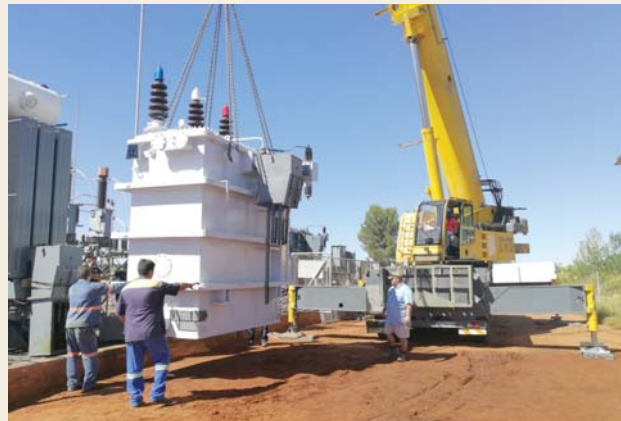
Hadison Park Substation – Replaced faulty transformer
